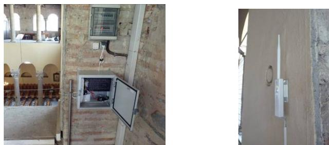
Figure 2: The WiFi installation inside the Monument. The equipment was placed so that it cannot be seen by visitors.
